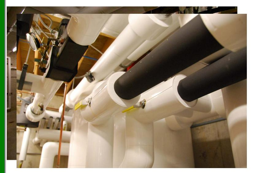
Super insulate hot water runs to minimize heat losses.
