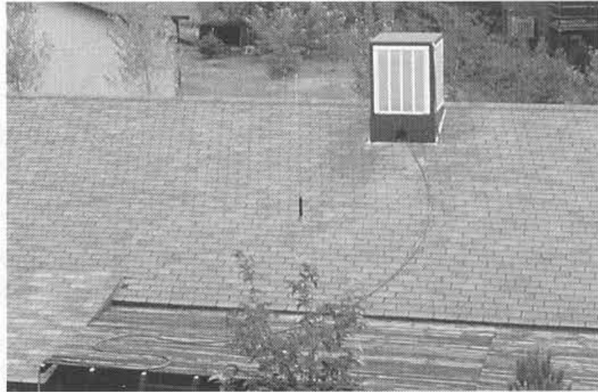
Figure 10.11b Evaporative coolers are widely used in hot and dry regions. This is an example of a direct evaporative cooler on the roof of a house.
