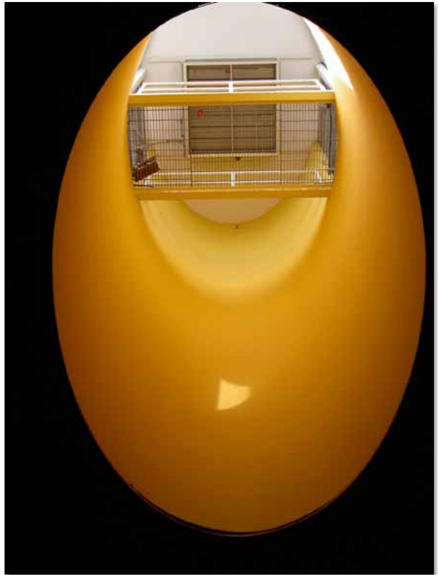
Solar chimney at the computer building, York University
