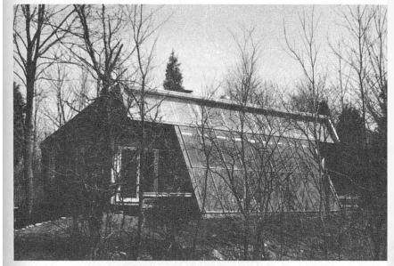
Figure 10.6: Solargreen exterior showing south-facing sunspace.
