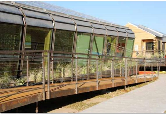
Arizona's house at the 2009 Solar Decathlon used a trombe wall made from water. Water has a high thermal storage capacity and is very "portable".
