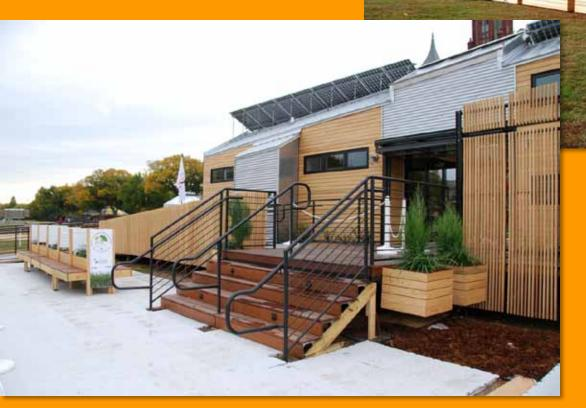
North face has small openings to minimize heat loss.
