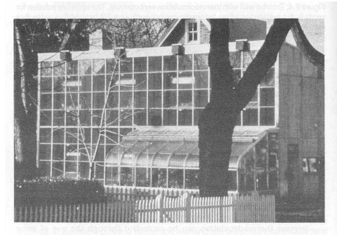
Figure 9.5: Kelbaugh house showing south facade with Trombe wall. (Photo courtesy of D. Kelbaugh.)
